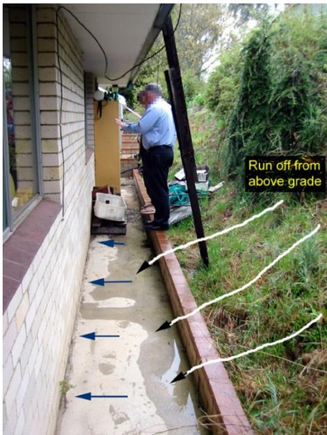
The site shown is a dwelling with a below grade slab. Water due to surface run off onto the surface, and also percolating ground water in through the base and edges have penetrated the slab and resulted in high moisture contents in the slab. A vinyl installation was put in place without a membrane and suffered de-bonding due to rising damp.
